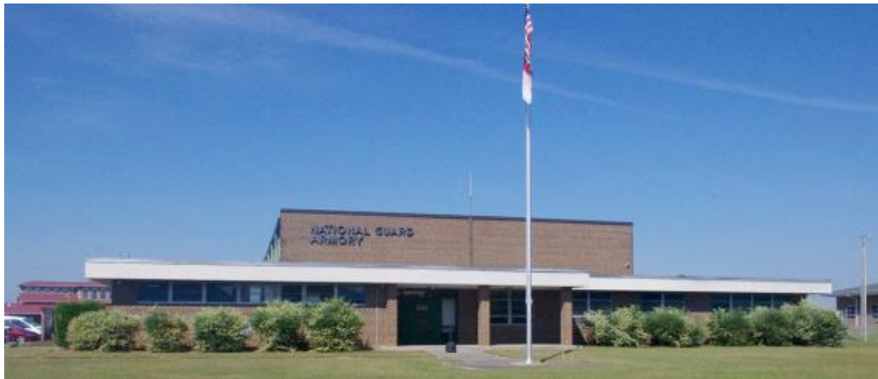
Figure 21. Façade of Type-D Armory in Greenville, North Carolina, constructed 1971 (Privett 2020: 38).
