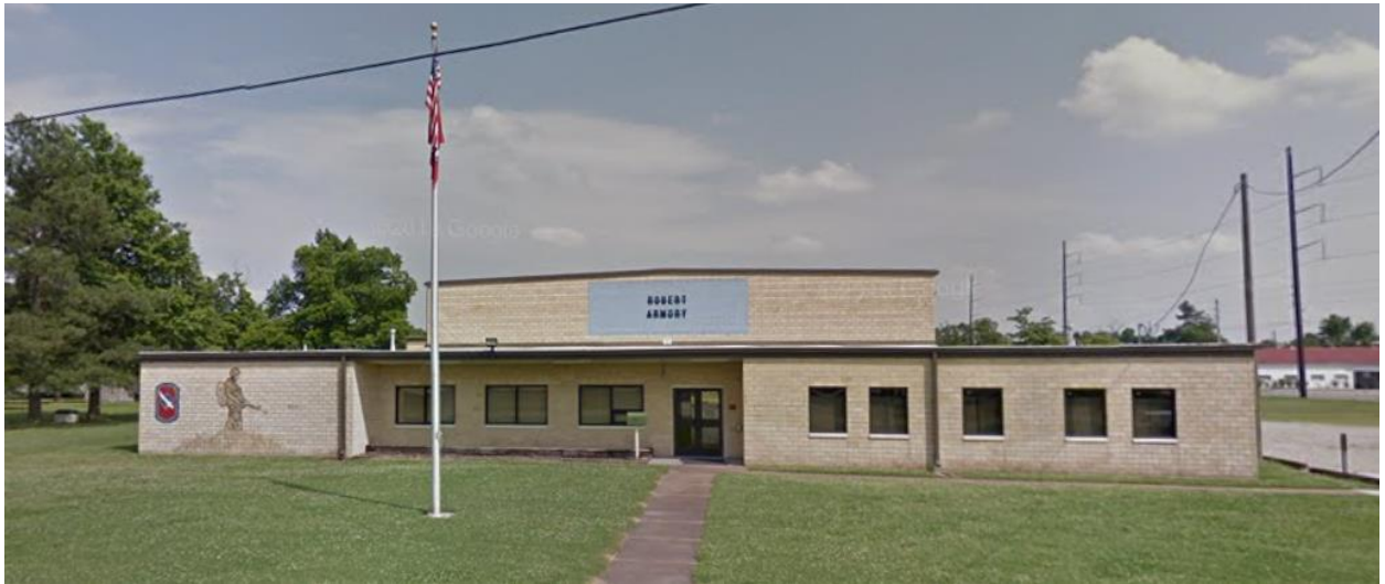
Figure 28. Façade of Type K Armory in Walnut Ridge, Arkansas (Google Maps 2019).
