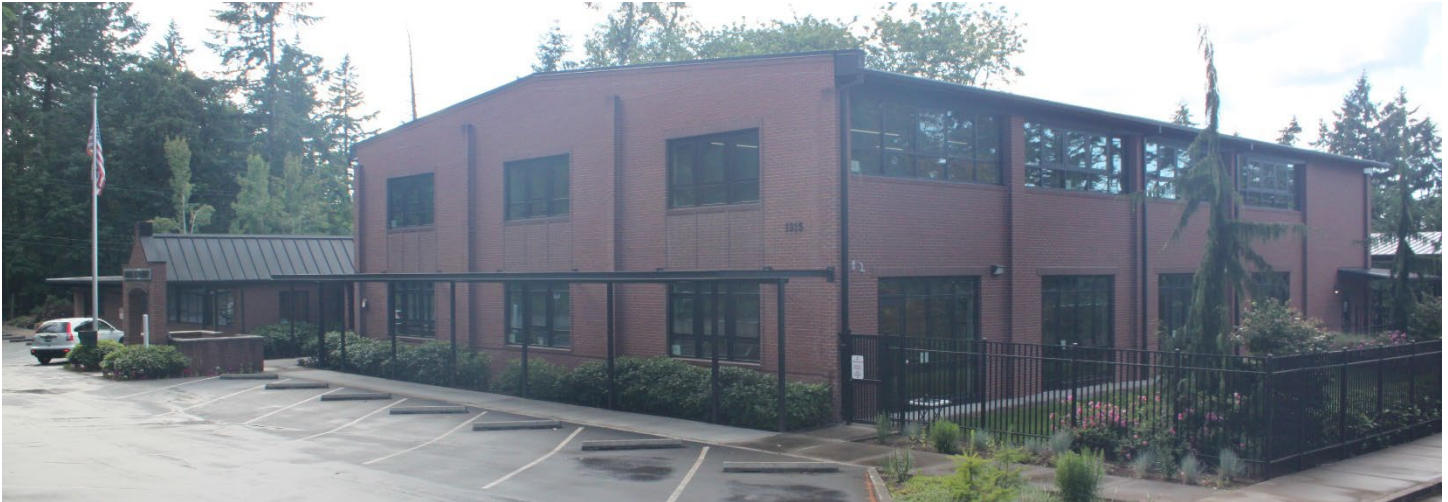
Figure 39. Current conditions at Lake Oswego Armory showing loss of integrity due to significant alterations in design, materials, workmanship, feeling and association (AECOM 2021).
