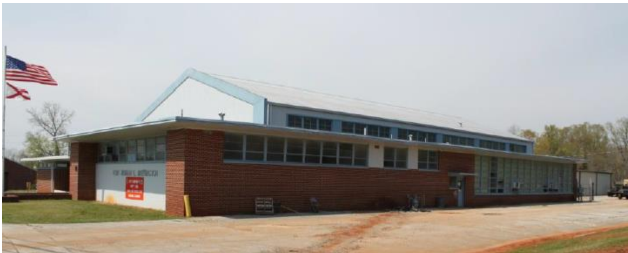
Figure 13. Oblique view of One-unit armory in Phoenix City, Alabama, constructed 1954 and designed by Evan M. Terry. In 2008, NGB consultants surveyed two armories of this plan type in Alabama and declared them as NGB Type B armories (Alabama Army National Guard archives, Burns & McDonnell 2008).
