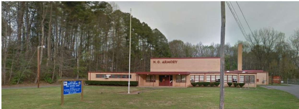
Figure 10. Type-Alt-A Armory, Belmont, North Carolina, constructed 1961 (Google Maps 2018).
