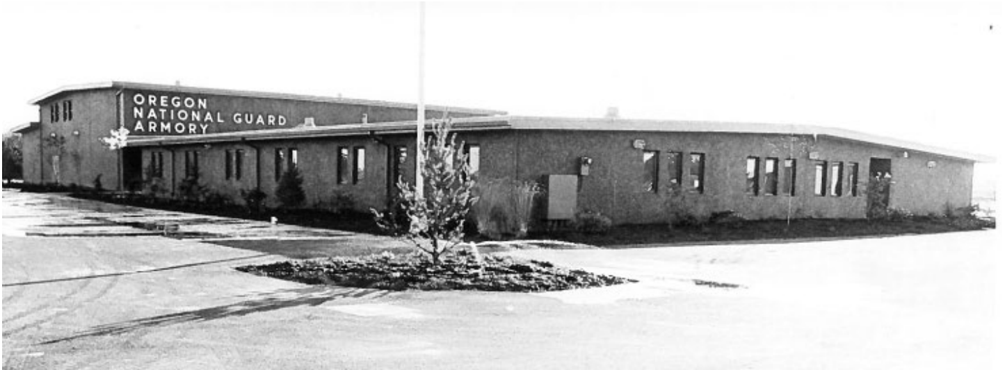
Figure 33. McMinnville Armory, ca. 1978 (Oregon Military Department).
