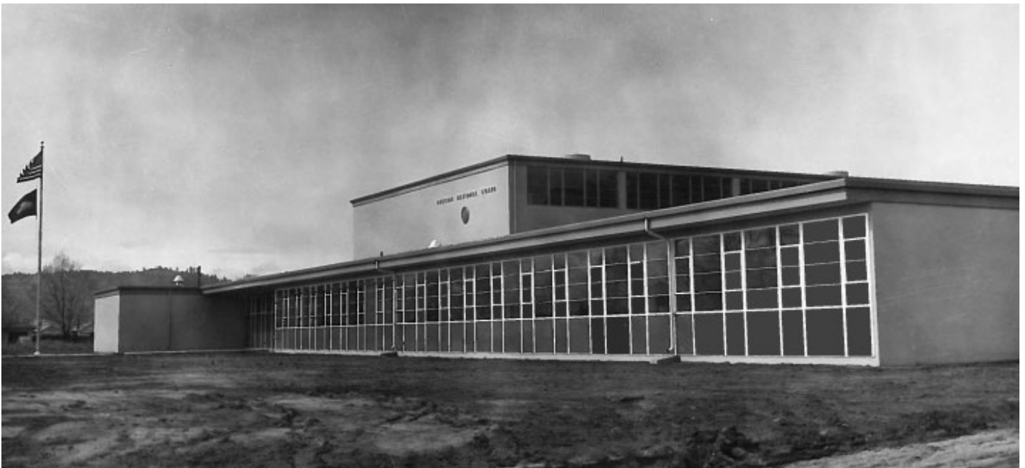
Figure 26: Klamath Falls Armory, ca. 1956 (Oregon Military Department).
