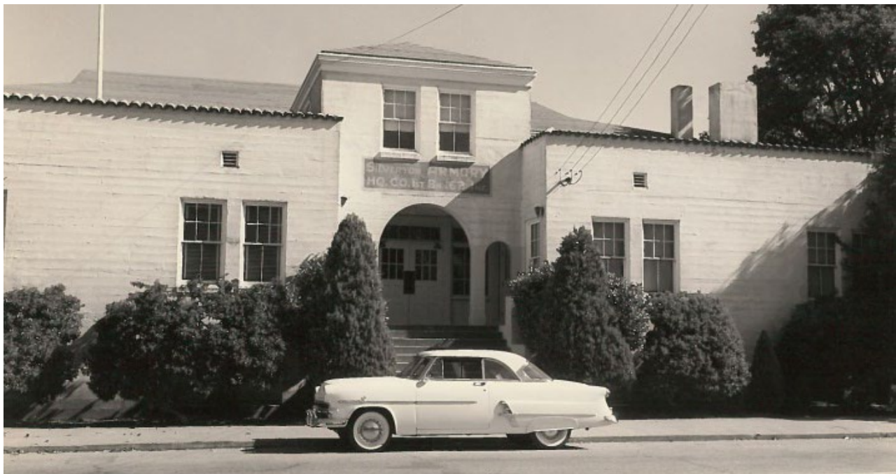
Figure 16. Revival Style Armory in Silverton, date unknown (Oregon Military Department).
