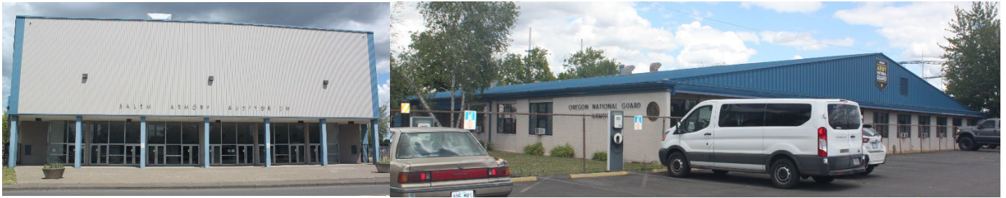
Figure 31. The Salem Armory is composed of two adjacent buildings: the Auditorium (left) and Armory (right) (AECOM 2021).
