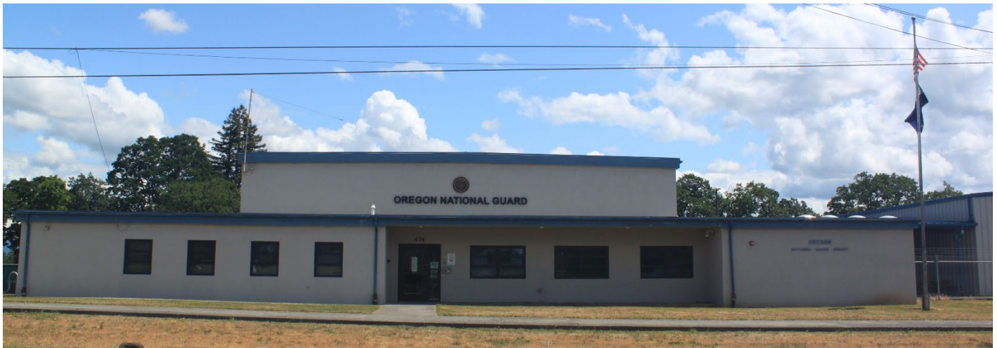
Figure 38. Current conditions at St. Helens Armory showing overall retention of integrity of design, materials and workmanship despite compatible window replacements (AECOM 2021).
