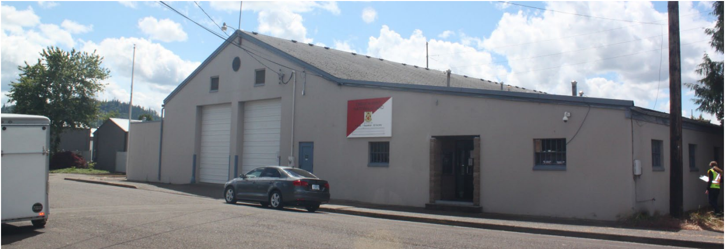
Figure 21. Current conditions at Lebanon MVS, the last of its type managed by OMD (AECOM 2021).
