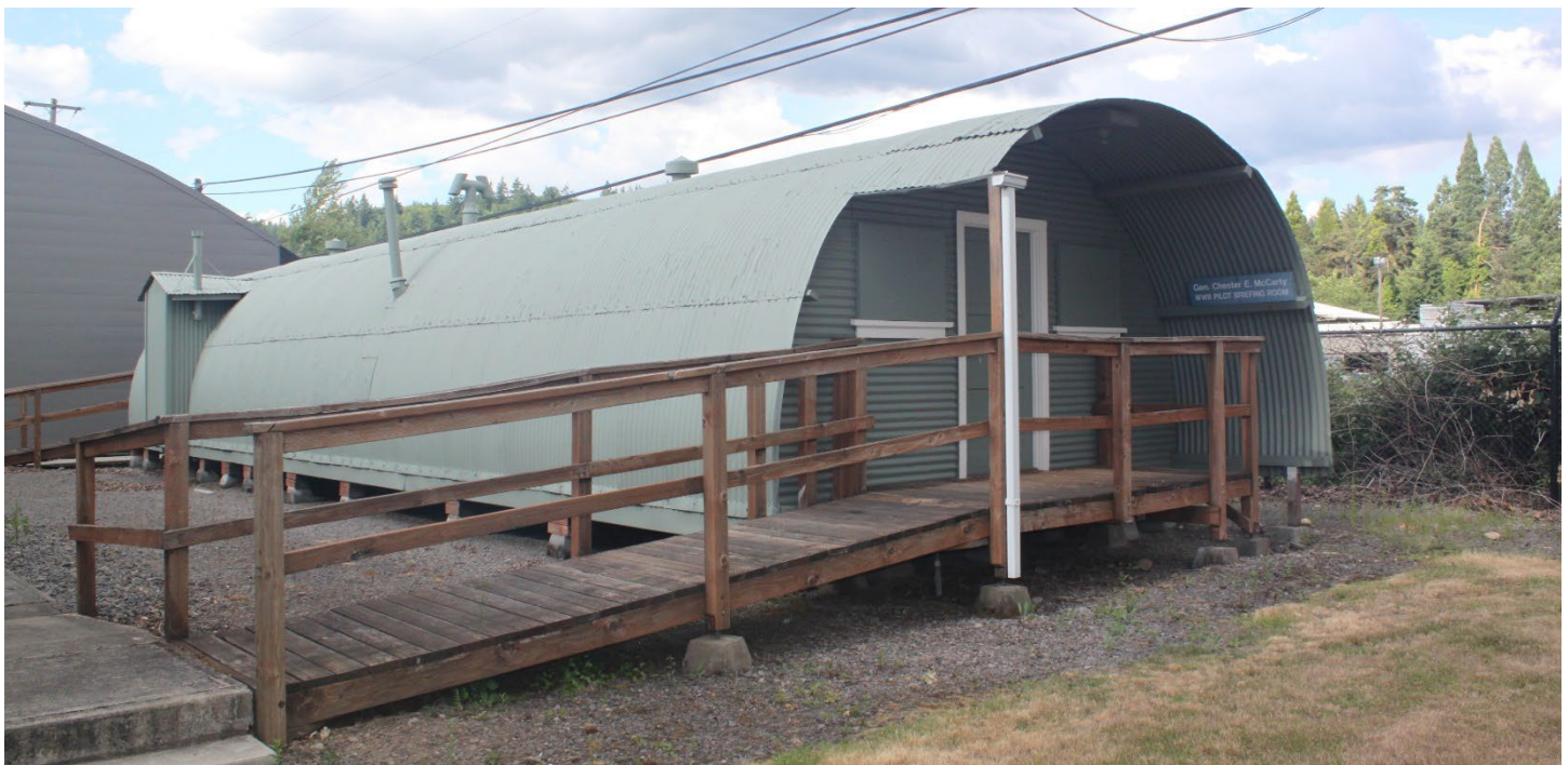
Figure 20. Small Quonset hut moved to Camp Withycombe to serve an interpretive function at the Oregon Military Museum (AECOM 2021).
