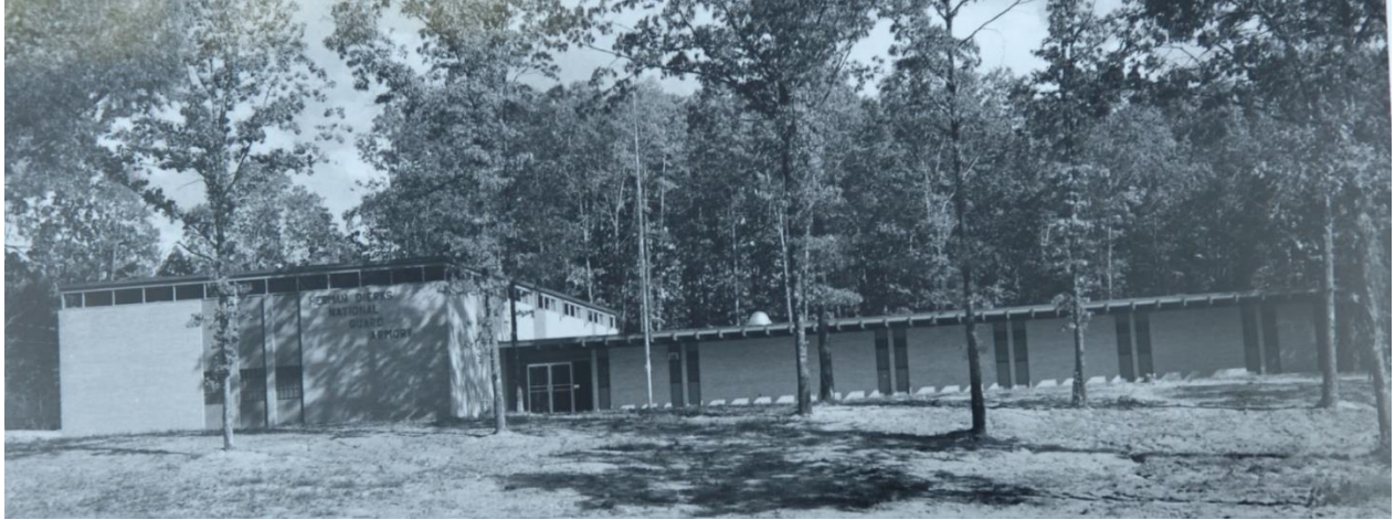
Figure 17. Façade of Type B-B armory, DeQueen, Arkansas, 1963 (Arkansas Army National Guard archives).
